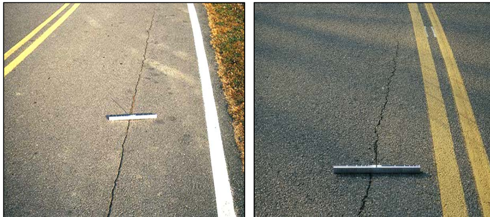
Figure 2.5: Longitudinal cracking measurements (Miller & Bellinger, 2014)
