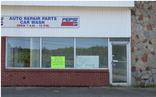
Fig. 2.7 $85,000 or best offer sign in window of vacant commercial building.
