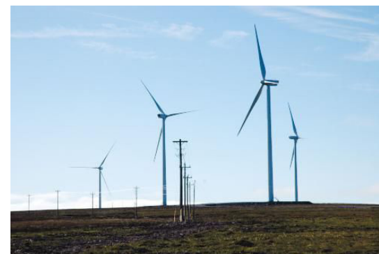
Fig. 2.24 Fermeuse Wind Turbines in Fermeuse, 90km from St. John’s. ( http://iwais.compusult.net/web/guest/optional-site-visits )
