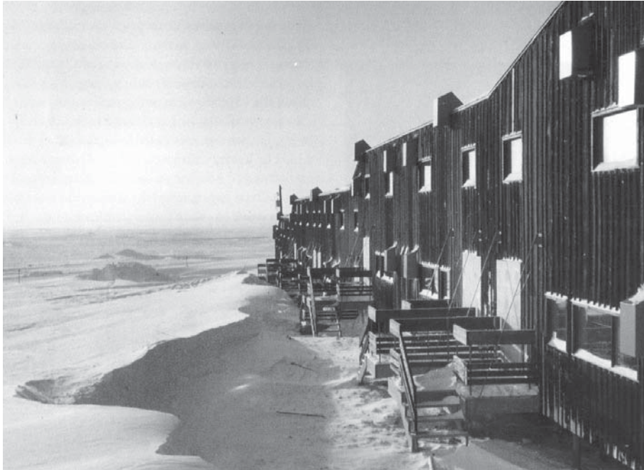
2.22 The completed terrace at Resolute Bay
