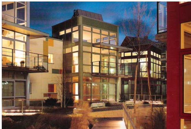
4.47 In the dark winter days, the lights of the interior living spaces shine outwards upon the exterior courtyard
