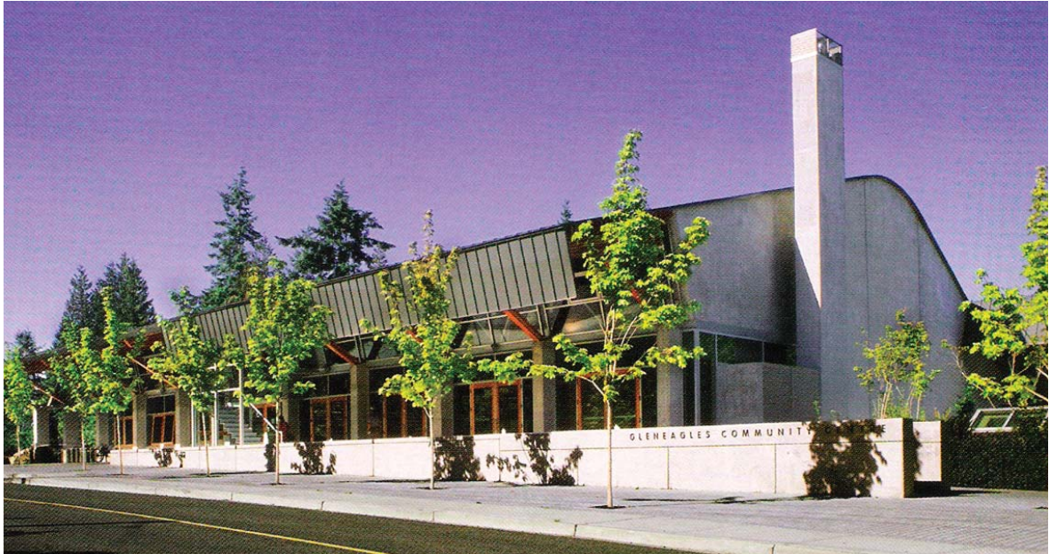
4.74 Gleneagles Community Centre, West Vancouver, British Columbia
