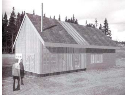
2.24 Semi-transparent fibreglass cladding in a three season space allows the play of light in the interior while promoting contact with the exterior landscape beyond
