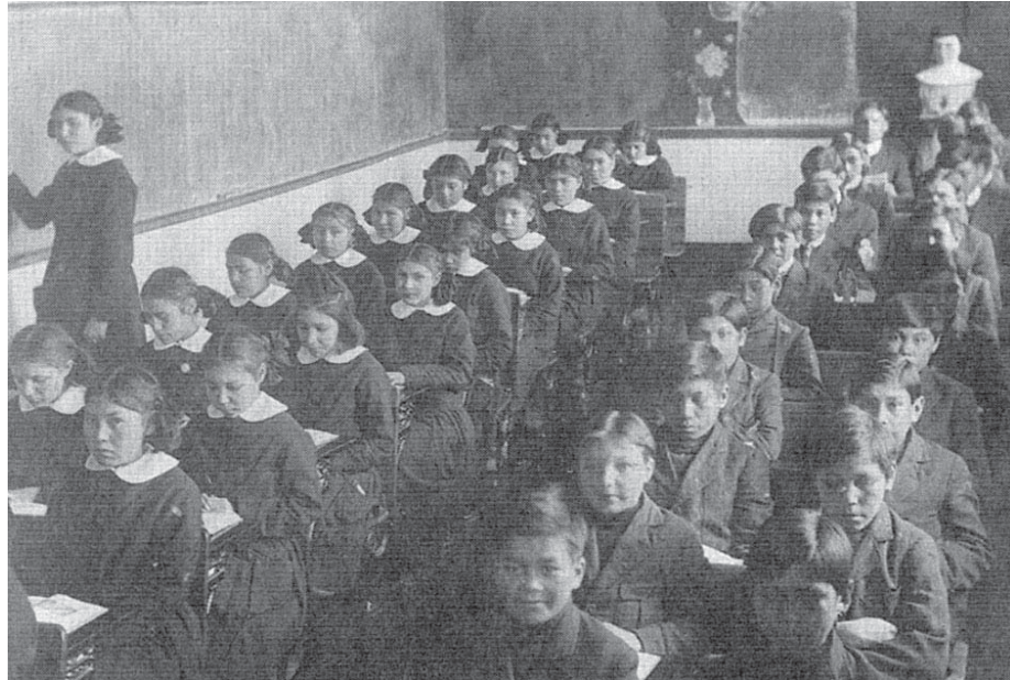
1.12 Residential School Classroom
