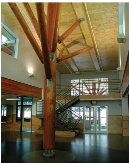
4.42 Main Foyer, Mayo Replacement School
